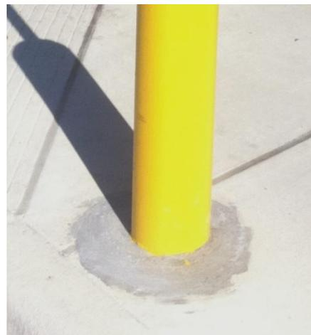
installation. Once the concrete is cored and the bollard is in place, the hole must be backfilled with concrete to secure the bollard. For added strength, these bollards are often filled with concrete, as well. Though the bollard pipe itself is relatively inexpensive, this installation method is costly and time consuming.
